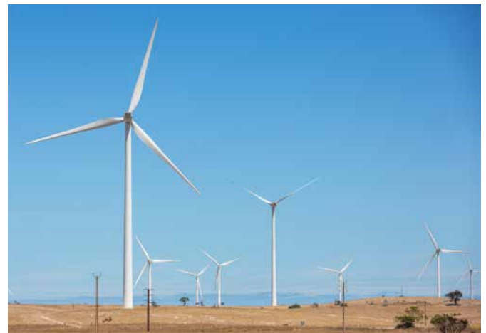
Lake Bonney wind turbine farm located in southeast South Australia
