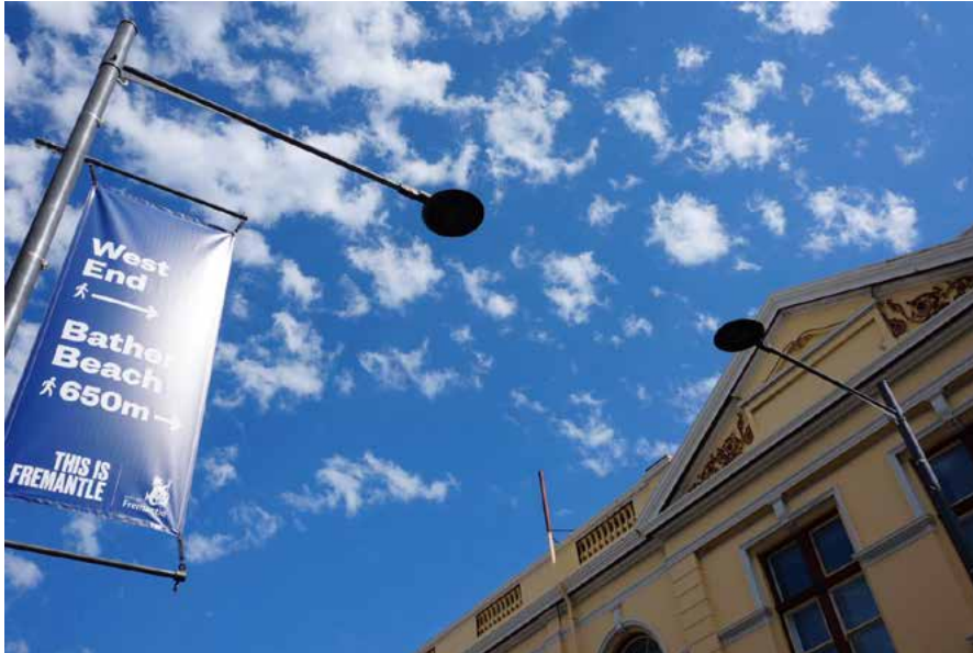
Figure 5.23: LED Street lights on Fremantle's cafe strip
