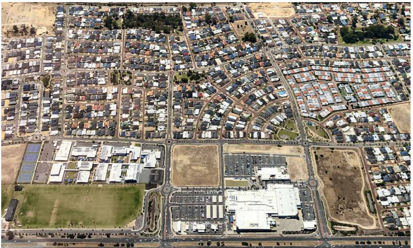
Figure 2.9: A new, treeless development in Perth's southern suburbs
