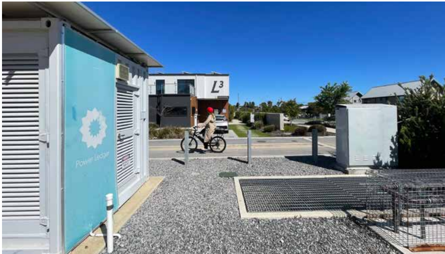
Figure 5.22: Residents of East Village at Knutsford have access to a shared battery
